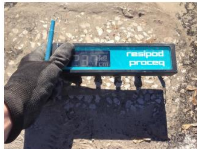
Figure 49. Surface resistivity testing on the bridge deck
