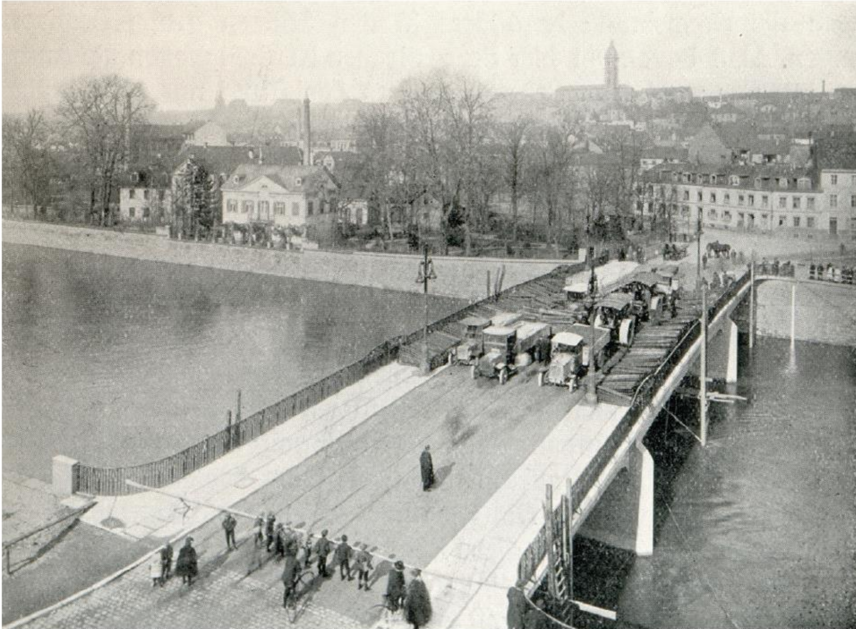
Figure 2.6 Proof load testing using enormous masses and loads (Mörsch, 1908)
