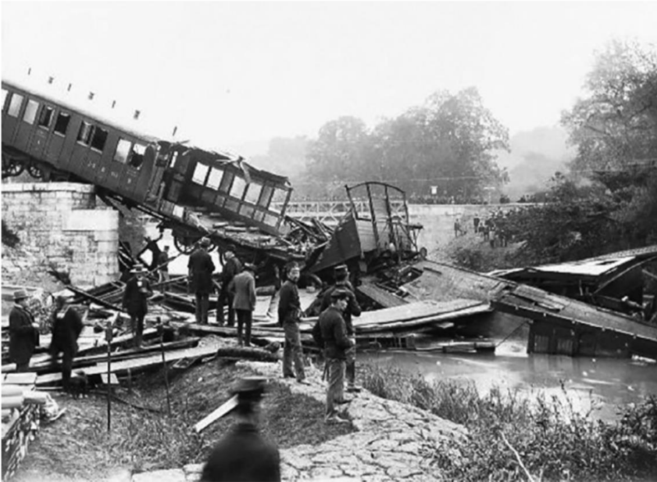
Figure 2.5 Picture of the bridge collapse in Münchenstein, Switzerland
